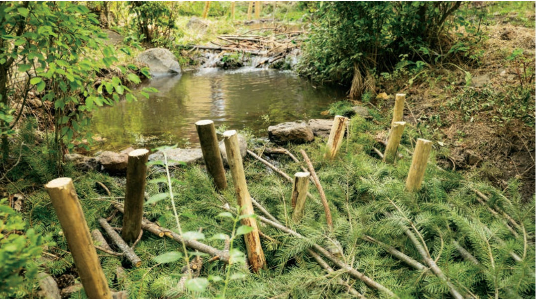
This beaver dam analog was built by crews from Anabranch Solutions in the summer of 2023, as part of their effort to restore stream processes and prepare the watershed for beaver reintroduction. Such human-made dams can entice beavers to areas that will benefit from their work. Credit: Sarah Koenigsberg
