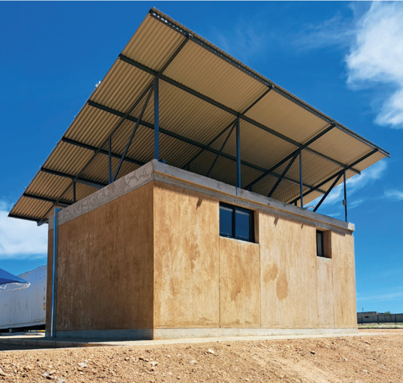
The first house constructed with mycomaterials demonstrates that it could be possible to build structures from in situ materials on the Moon and Mars. The illustration at left shows the building’s construction plan, while the top photo shows construction in progress. The photo above shows the final product, with mud plaster covering “mycoblock” walls capped with a concrete roof. On top sits a metal roof supporting solar panels. Credit: Mycohab Ltd.
