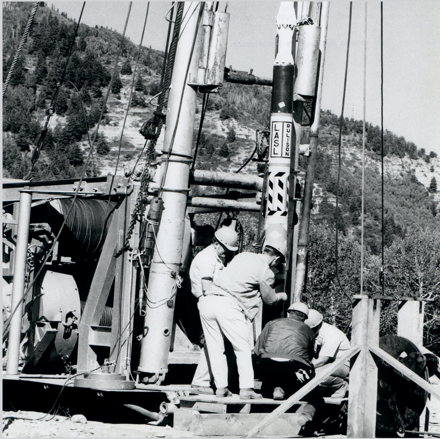
The Project Rulison 40-kiloton nuclear device, part of the AEC's controversial Plowshare program, proposed the detonation of a nuclear explosive deep underground in Colorado to stimulate the release of natural gas. It was lowered into its 8,442-foot deep emplacement hole on August 14, 1969. (DOE)
