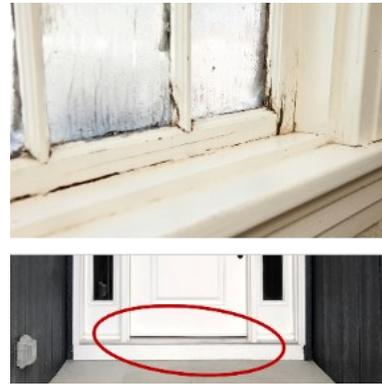
**Figure 8.** Example of cracks around a window and a gap under a door that may lead to leaks and infiltration of outdoor air.
