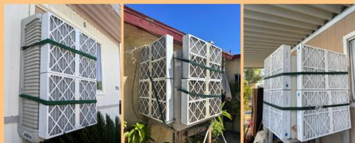
Examples of swamp coolers with MERV 13 rated filters attached. Photo credit: FRESSCA Study Research Team.
