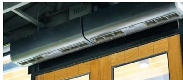
**Figure 10.** Example of air curtains installed above a door frame.
