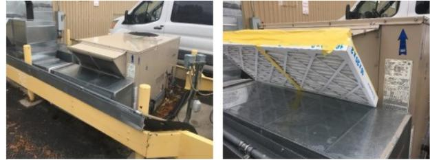
**Figure 7.** Images showing additional filters attached to HVAC air intake. Images from ASHRAE: Planning Framework for Protecting Commercial Building Occupants from Smoke During Wildfire Events.
