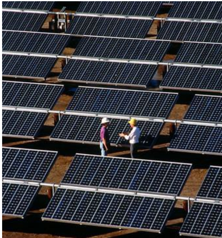
Figure 5.19-3. PV Panels in a Single-Axis Tracking System, Sacramento Municipal Utility District, Hedge Substation (Credit: Sacramento Municipal Utility District; Source: NREL 2009)
