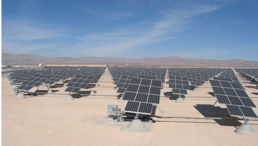
Figure 5.19-2. PV Panels in a Dual-Axis Tracking System, Nellis Air Force Base, Nevada (Credit: Argonne National Laboratory)
