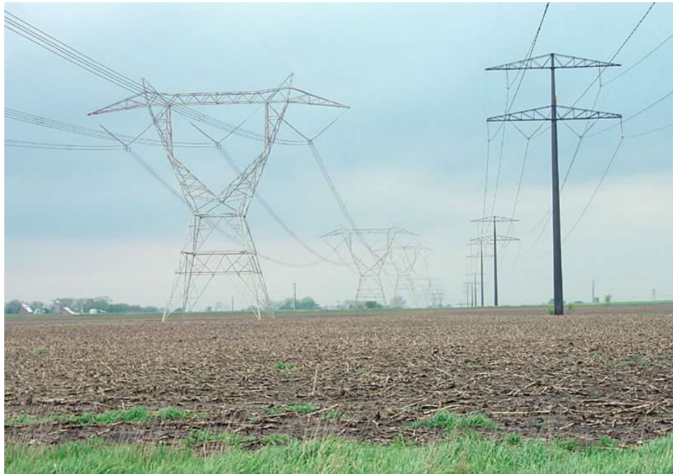
Figure 5.19-10. Lattice (left) and monopole (right) Transmission Towers (Source: Argonne 2007)
